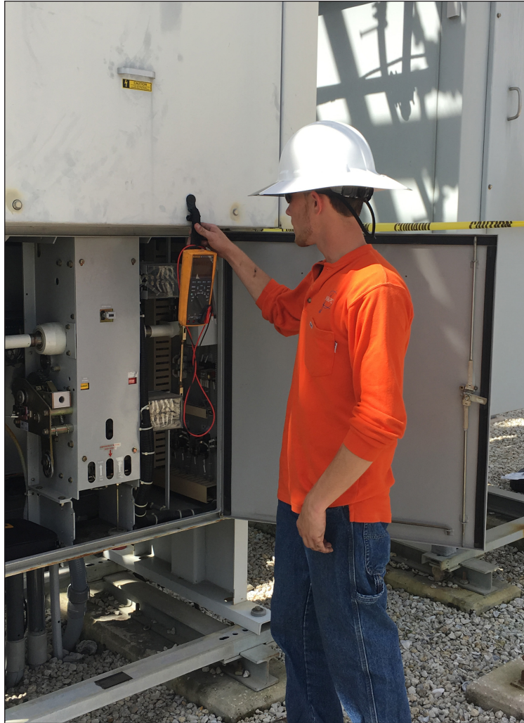
Ryan Collins, 22, checks a transformer to make sure the complex control system is operating correctly.
