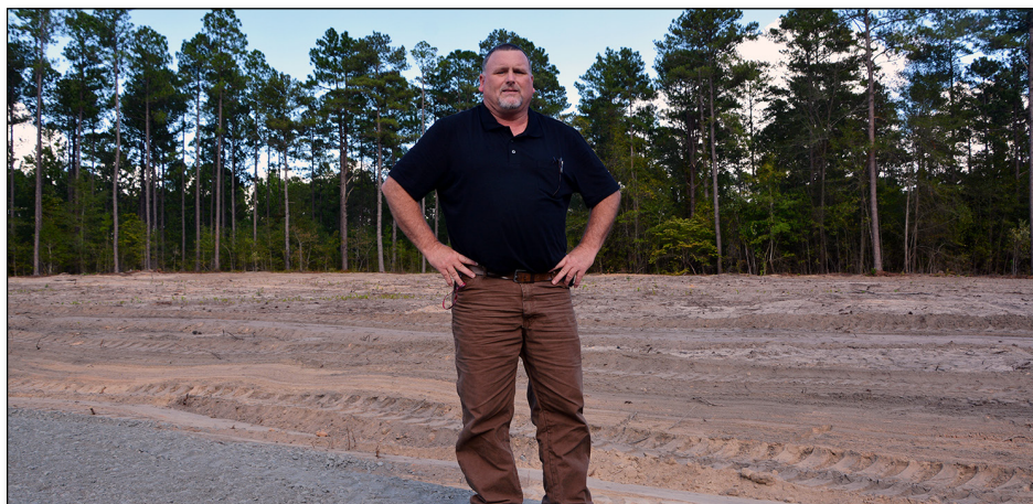
Scott Caulder stands in the area being cleared for Richmond Community College’s new Electric Lineman program.
