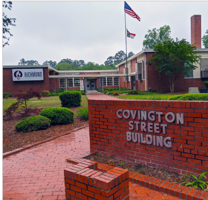
The Covington Street Building in Laurinburg is now a part of RichmondCC’s Scotland County Campus. The building houses the SEARCH program, as well as general college education classes.
